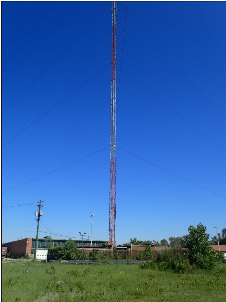
Figure 20. Communications facility, view looking southwest.
