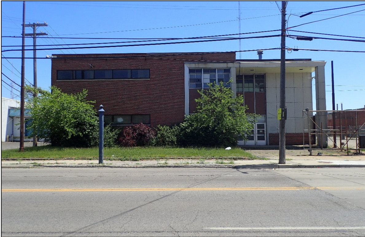
Figure 15. Building façade, view looking east.
