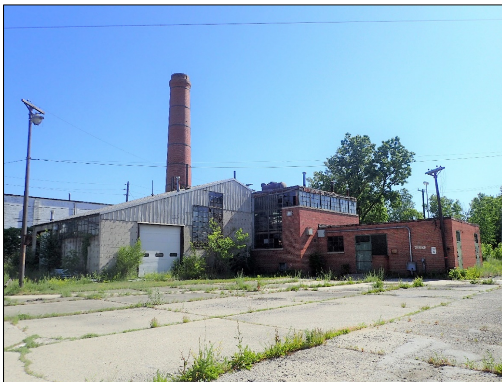
Figure 17. Heating plant, view looking northeast.
