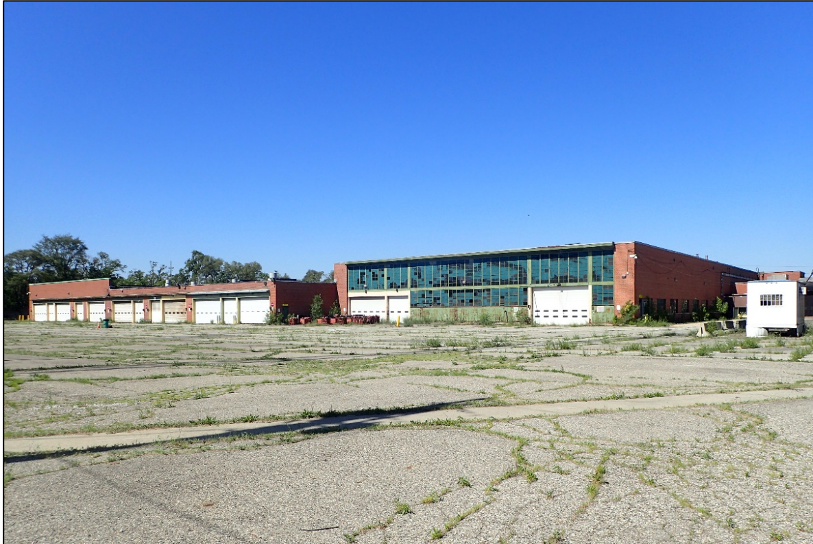
Figure 12. Coolidge Terminal, view looking southwest. At left is the storage wing, and visible at right is the maintenance wing. The bus washing wing is outside the frame to the right.
