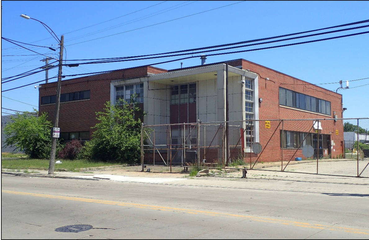
Figure 14. Coolidge Administrative Building, view looking northeast.
