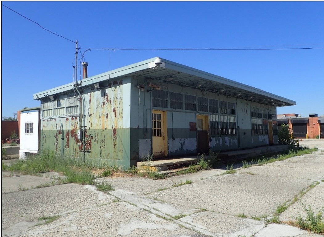
Figure 18. Fare Box House, view looking southwest.
