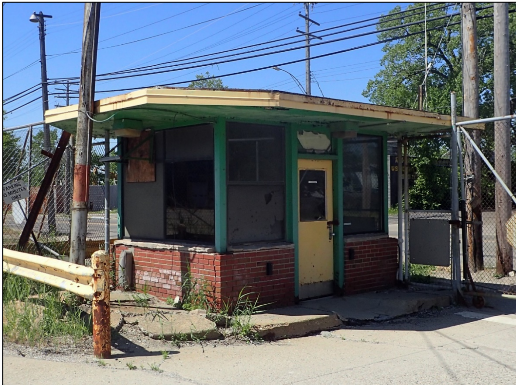
Figure 16. Gatehouse, view looking southwest.
