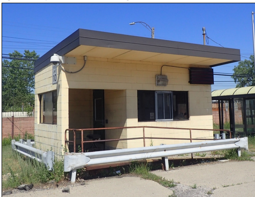
Figure 19. Dispatch House, view looking northwest.
